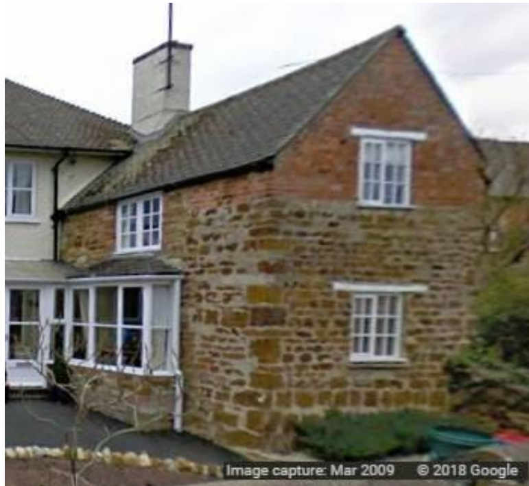
Photograph of the Farm Worker’s Cottage taken in 2009.
