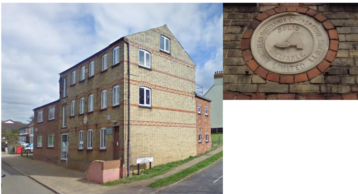
RSD43 – Britannia House, Denford Road, Ringstead
