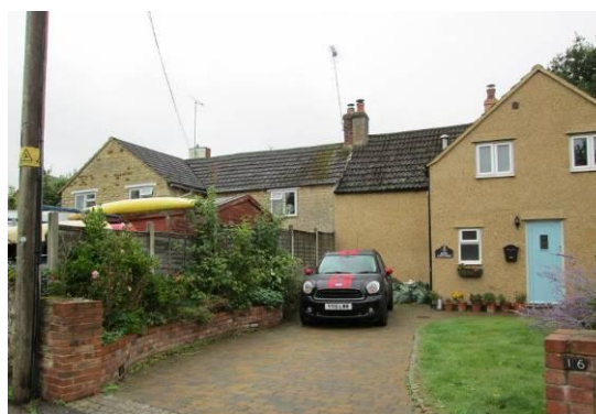
The 1838 cottage was originally a single rectangular stone building, some later extension work is evident and the rendering of No 16 hides the building fabric.
